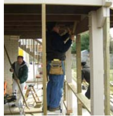
Our local RT team constructs the Briseno's screened-in porch
